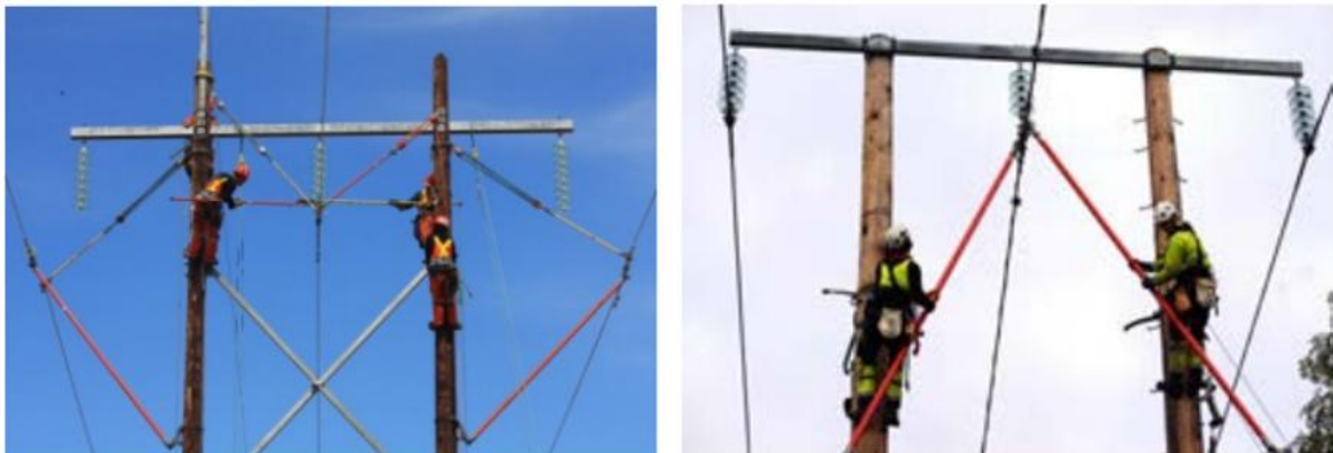
Figure 4 – Replacing insulators on a 132 kV power line [3]
